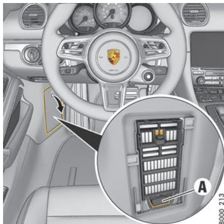
Fig. 75: Diagnostic socket in the fuse box in the left footwell
